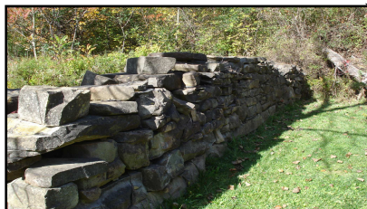
The foundations shown in this photo are rebuilt walls (using stones found at the site) on the visible foundations from the mills. These walls were rebuilt by Historical Society volunteers a few years back.
